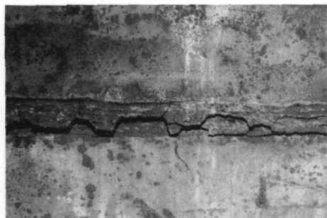
Figure 1 Cracks of FCCU.
