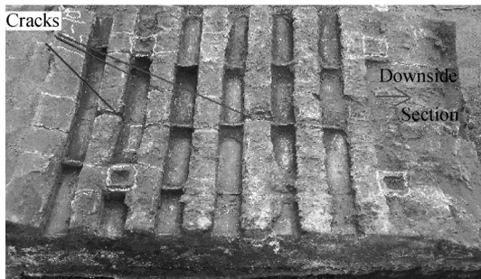
Fig. 4. Damage of the stave for BF.
